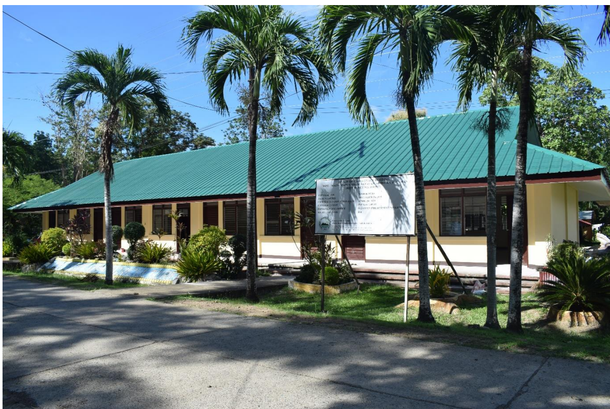
The newly repaired CAFES Office Building.
